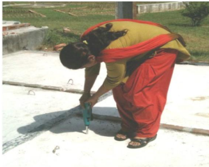
Fig. 3.13: Rebound Hammer Test
