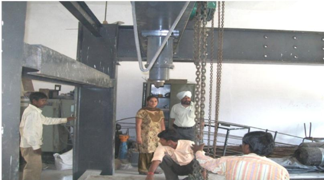
Fig.3.11: Work in Progress
