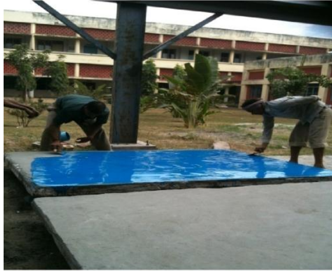
Fig.3.14: Application of Epoxy
