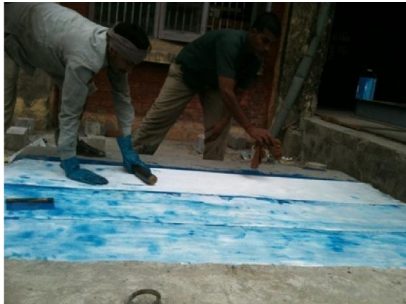
Fig.3.16: Rolling of GFRP
