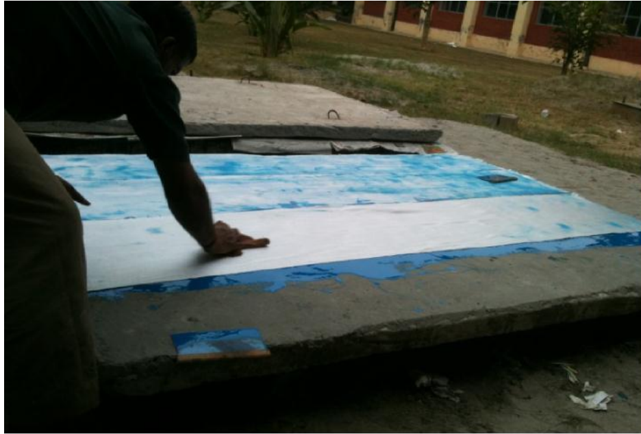
Fig.3.15: Placing of GFRP
