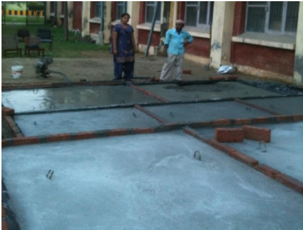
Fig. 3.7: Curing of slabs
