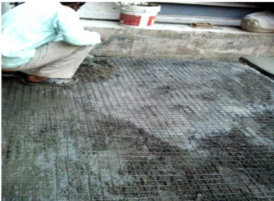
Fig.3.18: Retrofitting with Ferrocement
