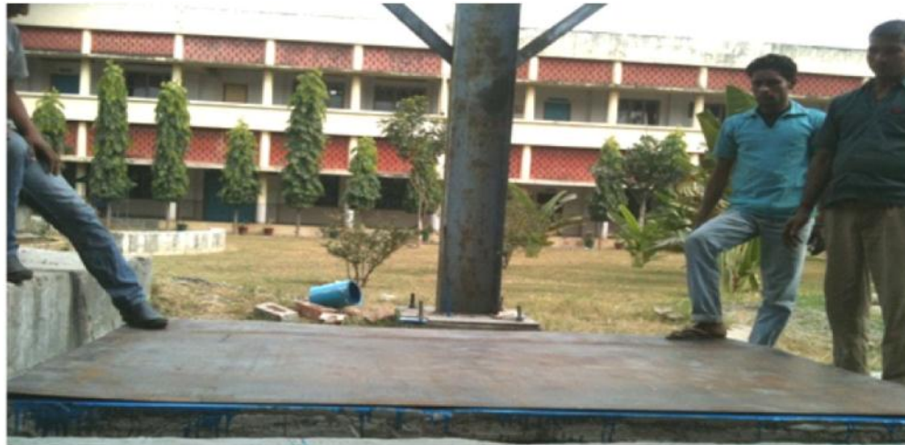
Fig.3.17: Placing of MS Sheet
