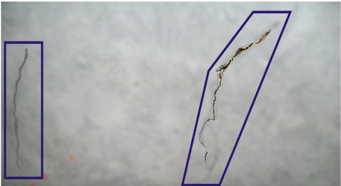
Fig.5.3: Development of cracks (typical)
