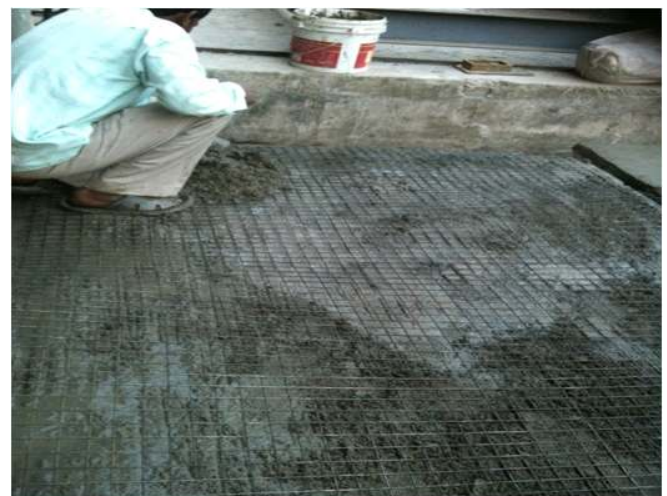
Figure 3. Ferrocement for Retrofitting
