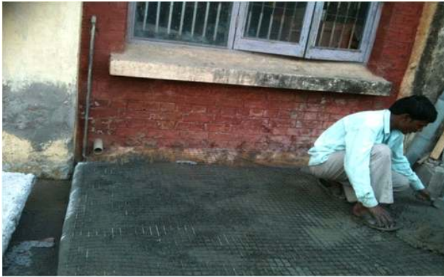
Figure 4. Placing of Ferrocement
