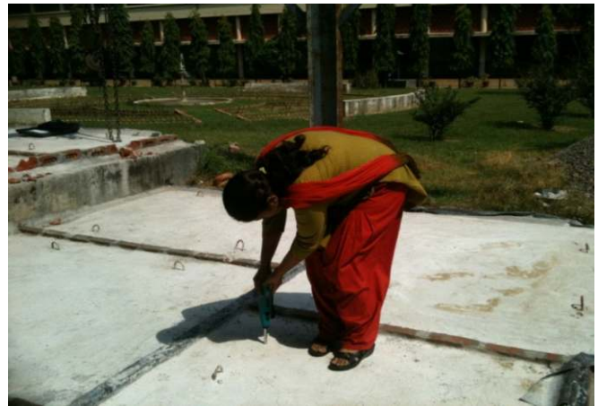
Figure 1. Rebound Hammer Test
