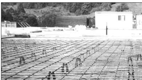
Figure 45: Project mesh simplifies mesh laps
