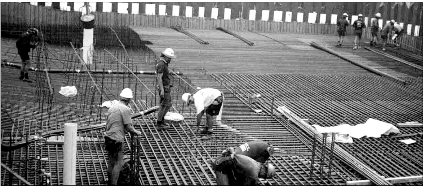
Figure 2: Reinforcement being tied on site
