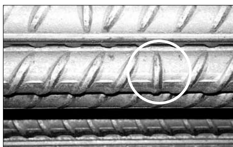
Figure 10: A vertical rib used as a mill mark
