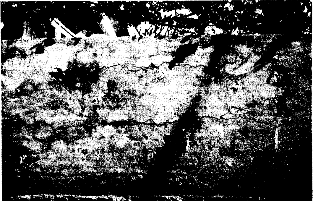
Photo 9 Horizontal Cracks in Compound Wall of Brickwork, having Horizontal Reinforcement; Brickwork being Exposed to Weather and Rain, Reinforcement has been Corroded, Resulting in Cracks; This Wall was Built in 1967
