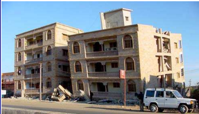
(b) 2001 Bhuj Earthquake
