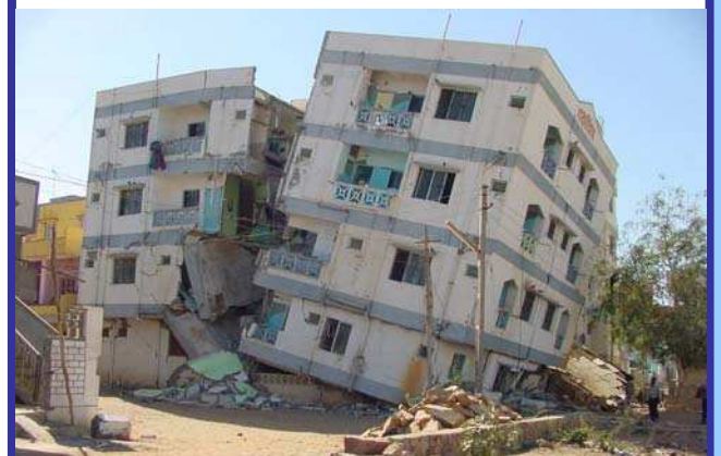
(b) Collapse of reinforced concrete columns (and building) during 2001 Bhuj (India) earthquake
