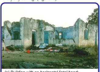
(a) Building with no horizontal lintel band: collapse of roof and walls
