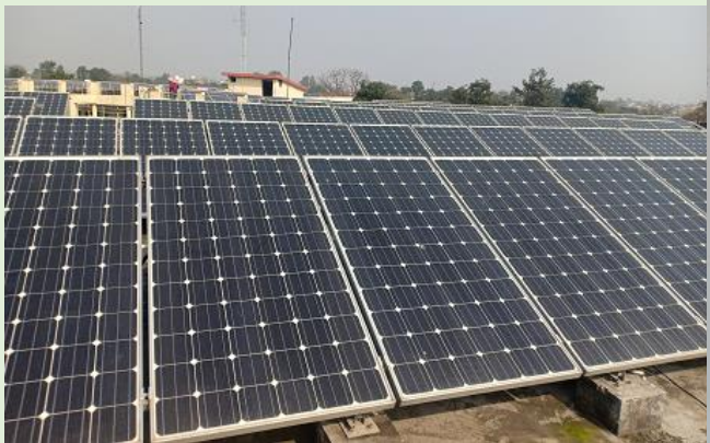
Fig: Grid Connected Solar PV plant on MBA block Rooftop (50+50kWp)
