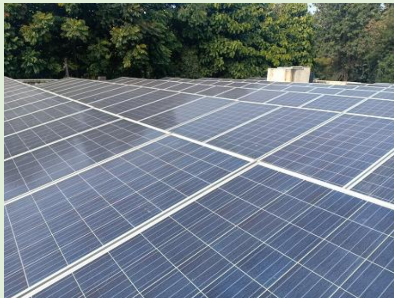
Fig: Grid connected Solar PV Plant on Administrative Block
